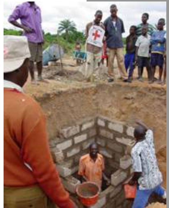
Building a latrine Photo: International Federation
